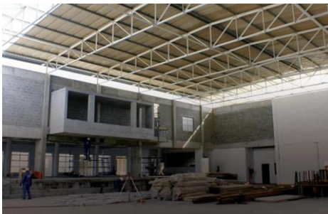
Over Purlin Plasterboard Industrial
