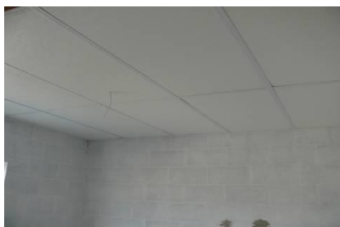
Retrofit H-Section Ceiling Vinyl Faced Board 600mm x 1200mm Office
